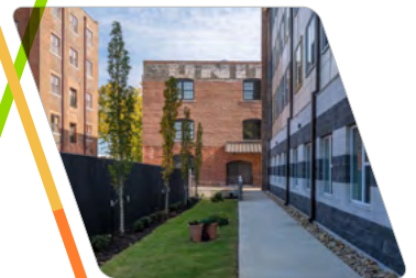
South Main Artspace Lofts in Memphis, Tennessee.
